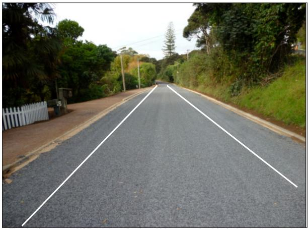
Nore: The edge line areas are NOT cycle lanes. Passing vehicles may need to drive in the edge line area when passing
