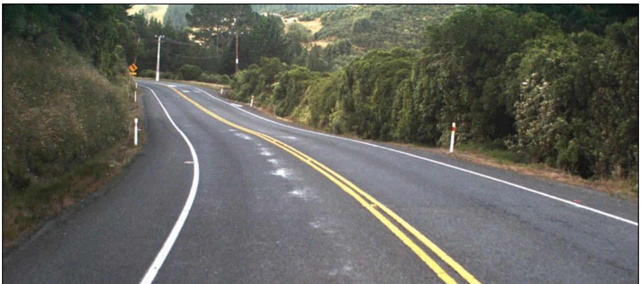
Figure 3-4: Approach to the short straight between the two left hand curves in the ‘broken back’ alignment heading west (Increasing RP 0/2.58)
