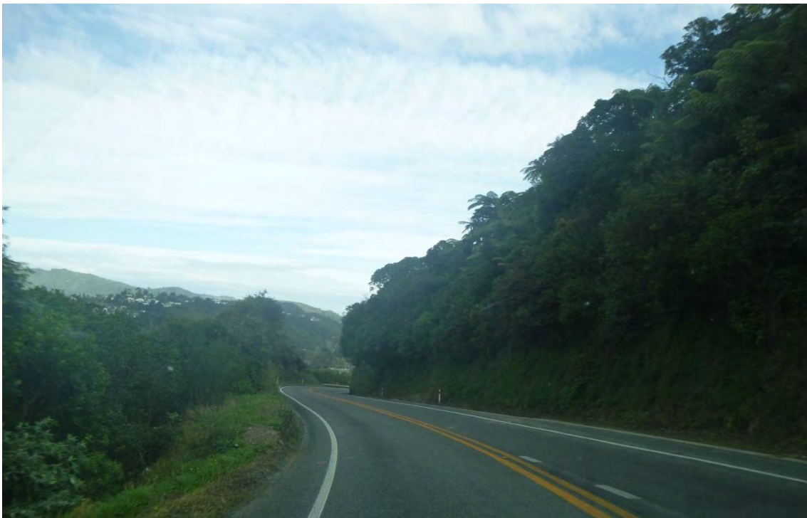
Photo 2: Narrow shoulders and out of context reverse curves, heading east
