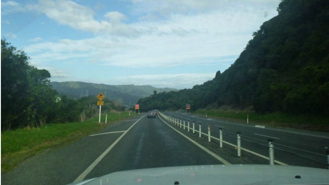
Photo 3: Existing wire rope barrier, heading east
