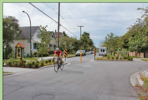
Example of treatment preventing ‘rat running’ along a neighbourhood greenway (Paul Krueger)
