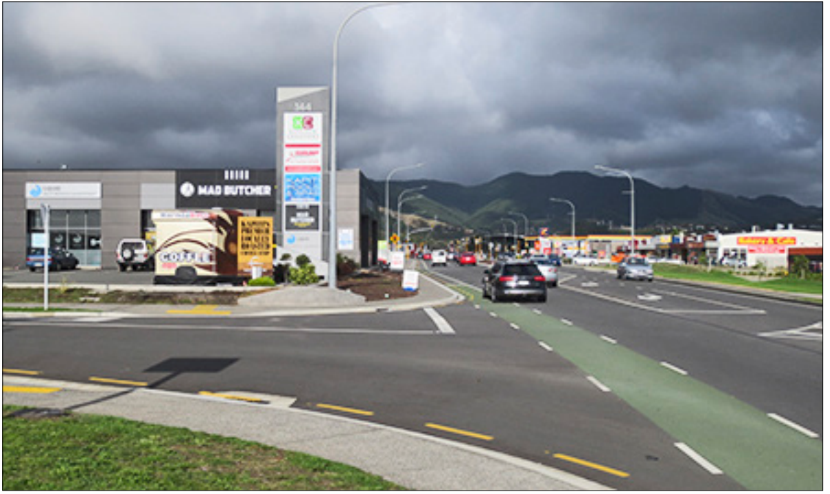
Encroachment onto future road reserve on Kapiti Road
