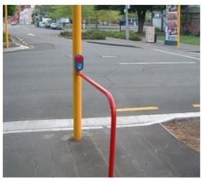
An example of an automatic bicycle detector call box, Christchurch, with detector loops underneath (note the hold-rail for waiting too)
