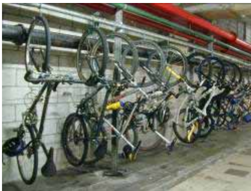
Photo 6: NZ Post bike rack with plastic covered hooks and horizontal plastic covered locking cable.
