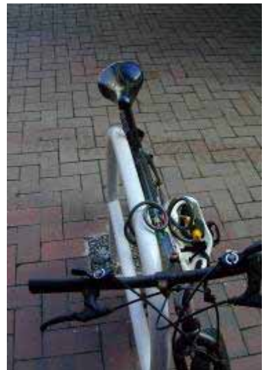
Photo 2: Metal to metal contact on Framescraper bike racks outside Wellington Railway Station.
