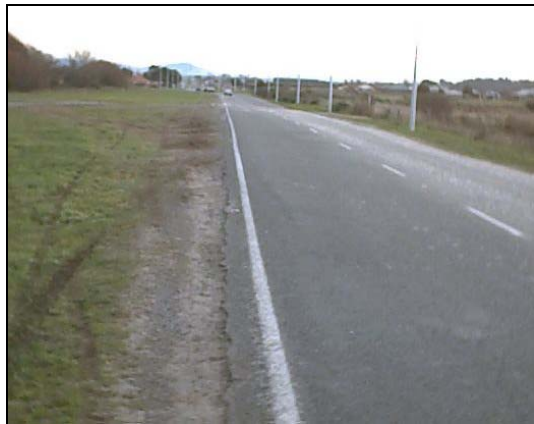
Figure 1: No shoulder, 70 km/h speed limit, 10,000 veh/day – cycling permitted.
