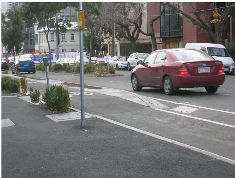
Figure 4.7: Kerb separated bicycle lane
