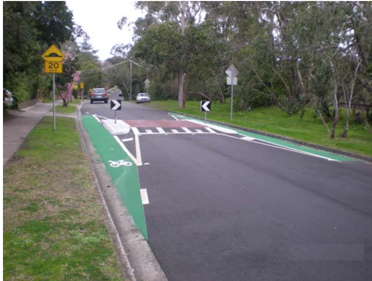
Figure 4.11: Example of good practice – cycle bypass of a road hump
