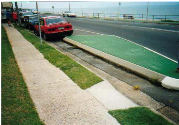
Figure 4.12: Parked vehicle blocks cycle bypass
